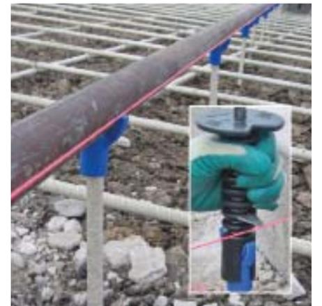
The Mako Screed Support System maintains the finished elevation of concrete,
