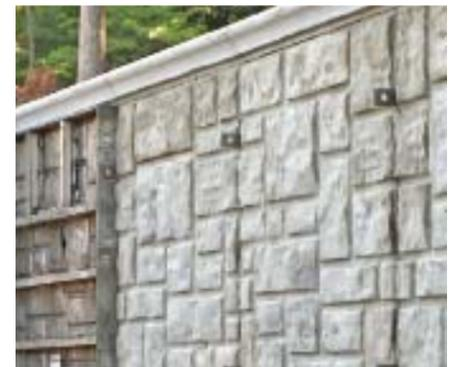
The all-aluminum ashlar stone concrete form uses an advanced stamping method that allows the aluminum sheet to be stamped in a deep ashlar-stone pattern. The result is a natural looking ashlar pattern without the need for formliners. The ashlar stone forms are compatible with any aluminum forming system.
